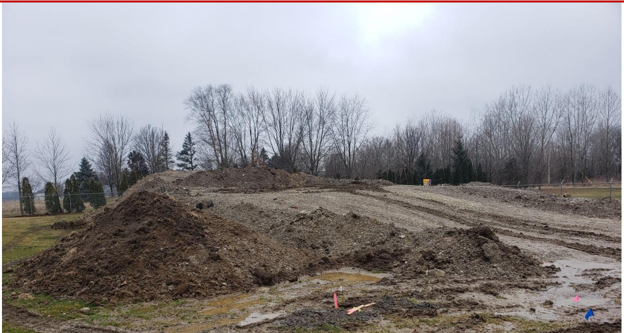
Photo 8: Topsoil stockpile to the left of stockpile
